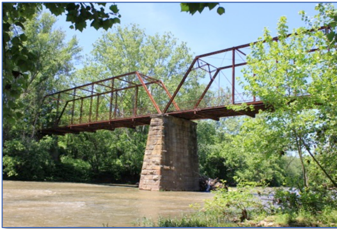
Shiloh Bridge Replacement, Tyler Co., WV Section 106 review and mitigation
