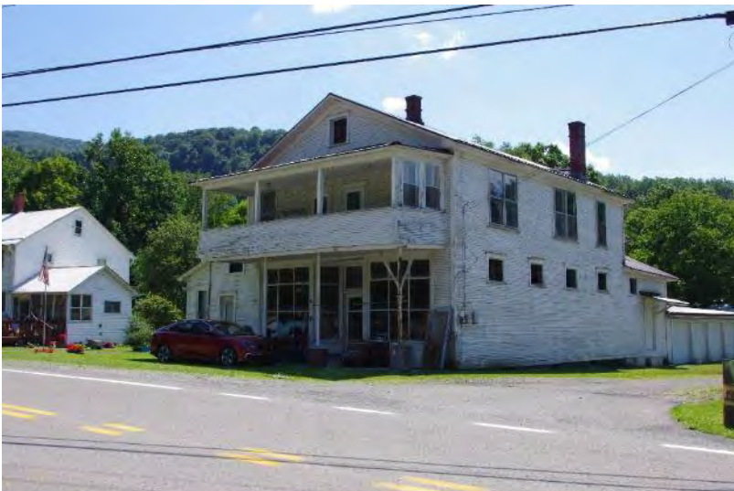
Otter Creek Boom and Lumber Company Store, one of the few early 20 th -century industrial buildings remaining in Hambleton
