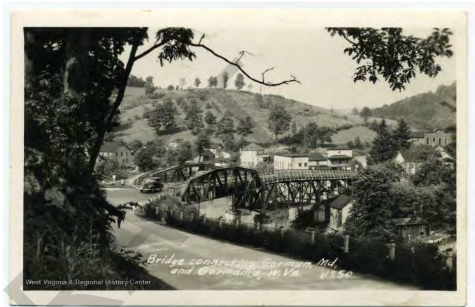
FIGURE 8. US ROUTE 50 (NORTHWESTERN TURNPIKE) BRIDGE OVER THE NORTH BRANCH AND WVC&P/WESTERN MARYLAND RR AT GORMAN, CA. 1930. (WV HISTORY ON VIEW)
