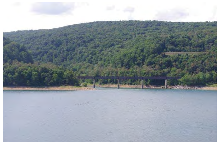
Railroad bridge on the post-lake alignment
