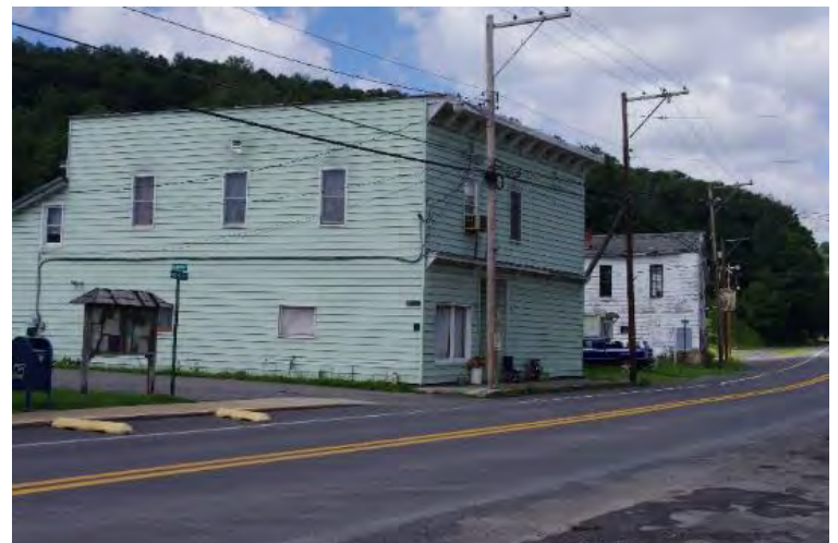
Commercial buildings across from railroad
