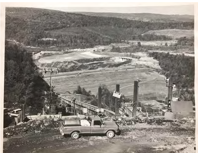
Jennings Randolph Lake (Bloomington Dam) under construction
