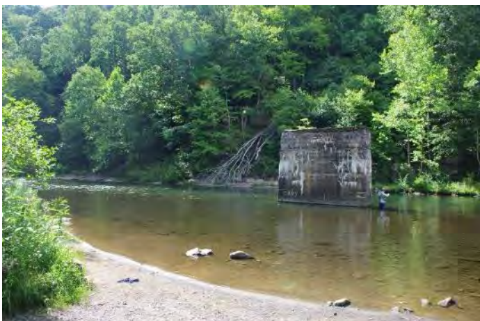
Former coal tram/conveyor pier
