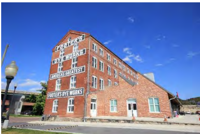
Footer Building (1906) Adaptive Reuse project
