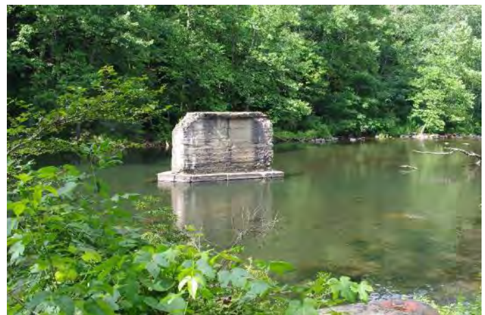
Former vehicular bridge pier
