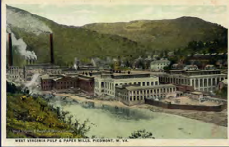
WEST VIRGINIA PULP & PAPER MILLS, PIEDMONT, W. VA.
