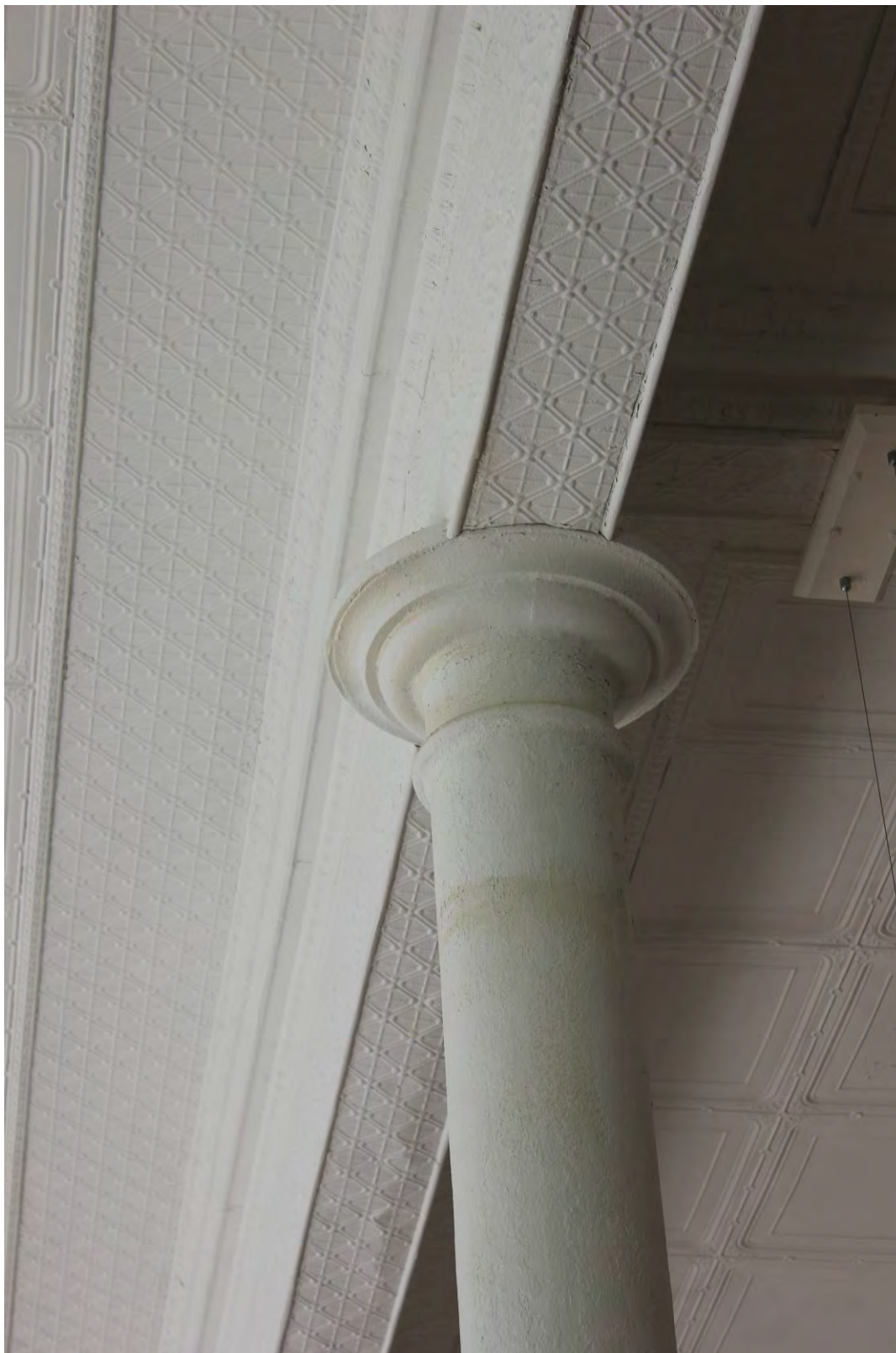
Photo #9: Interior: Metal column and stamped metal ceiling in main retail space, first floor
