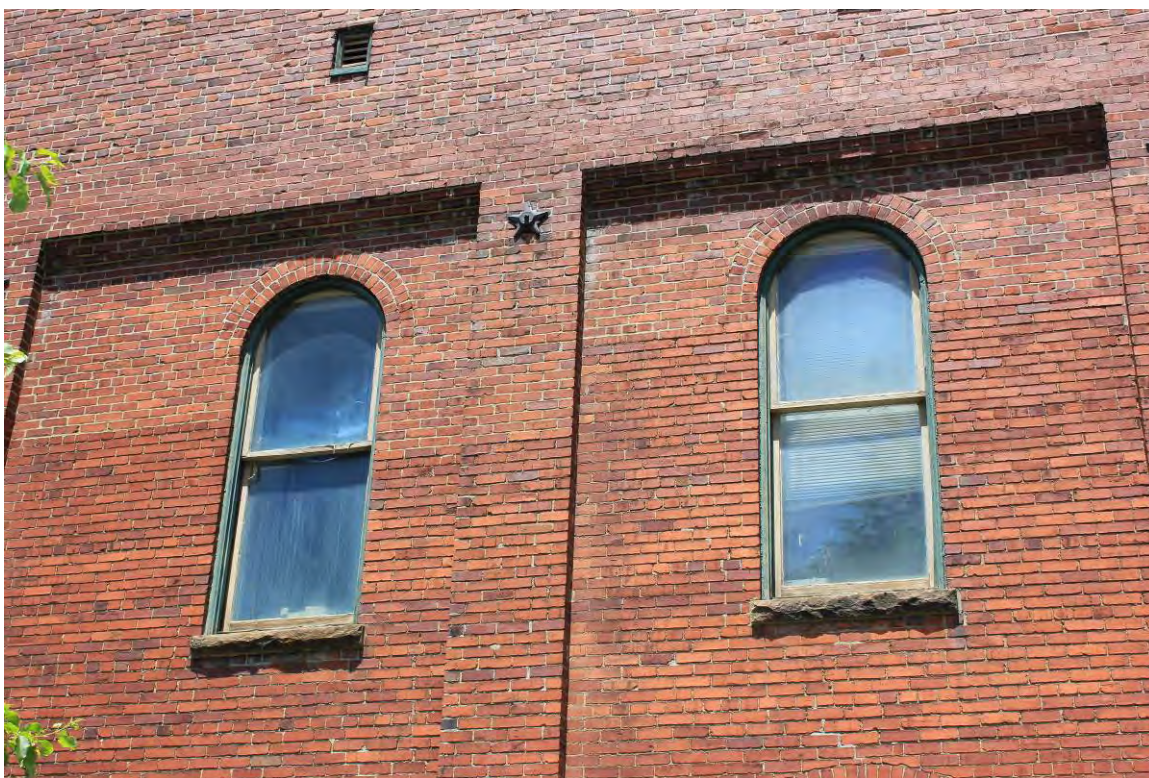
Photo #7: Detail: Arched sash windows and star tie rod anchor on south elevation
